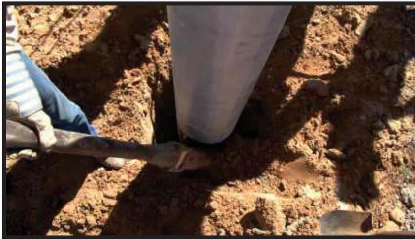
*Figure 3-12: Crewmen Tamping Backfill Around Pole Base*
