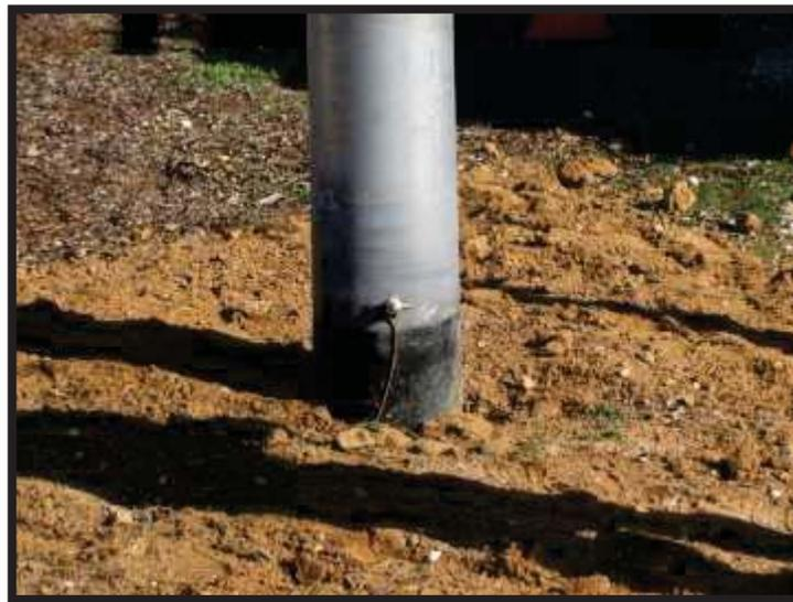
*Figure 3-15: Pole Base Ground Lead*
