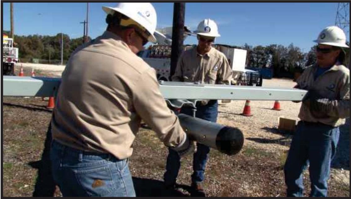
*Figure 3-4: Workers Installing an FRP Crossarm*
