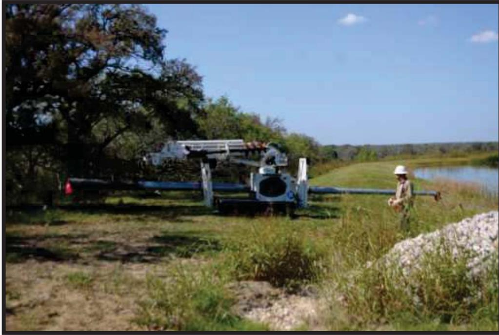
*Figure 3-13: Steel Pole Being Carried by a Remote-Controlled Mini-Derrick*
