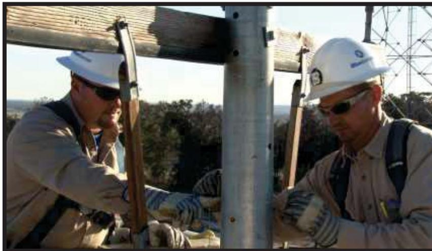
*Figure 3-8: Lineworkers Marking the Second Hole Using the “String” Method*
