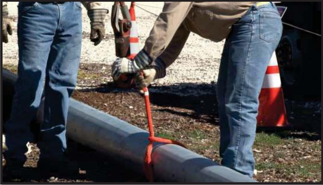
*Figure 3-10: Rigging the Steel Pole for Lifting*
