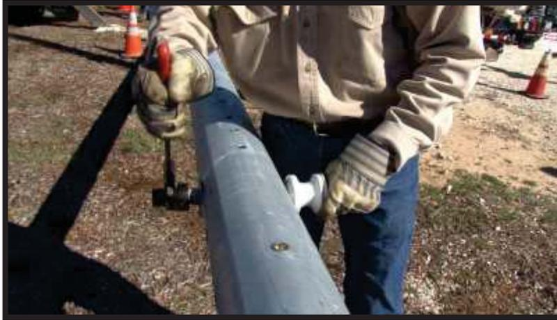
*Figure 3-5: Crewman Tightening Bolt “Snug Tight”*
