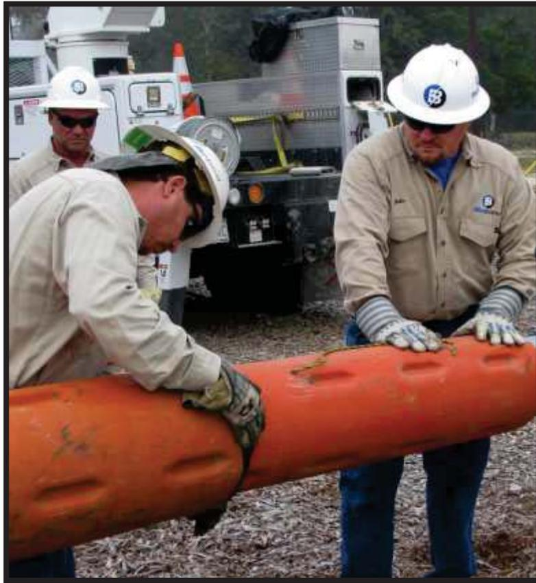
*Figure 3-16: Insulating Pole Guard Applied to the Steel Pole*
