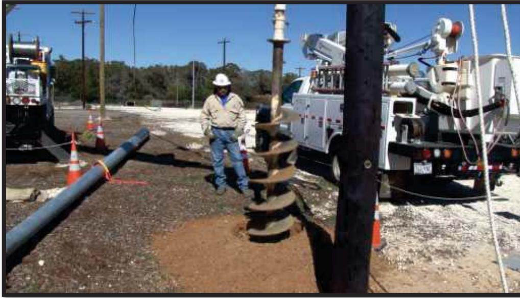
*Figure 3-9: Crew Digs the Hole for the Steel Pole Direct Embedment using Digger Derrick*
