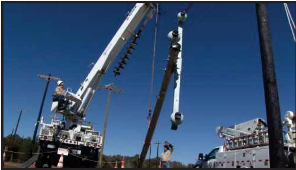
*Figure 3-11: Digger Operator and Ground Worker Maneuvering Pole*
