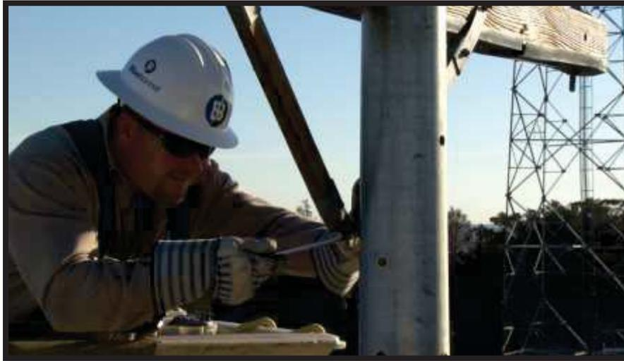
*Figure 3-7: Lineworker Marking the First Hole to be Drilled*
