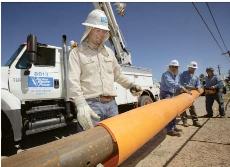
Crew installs cover-up over the steel to provide protection in case of accidental contact with an energized line.
