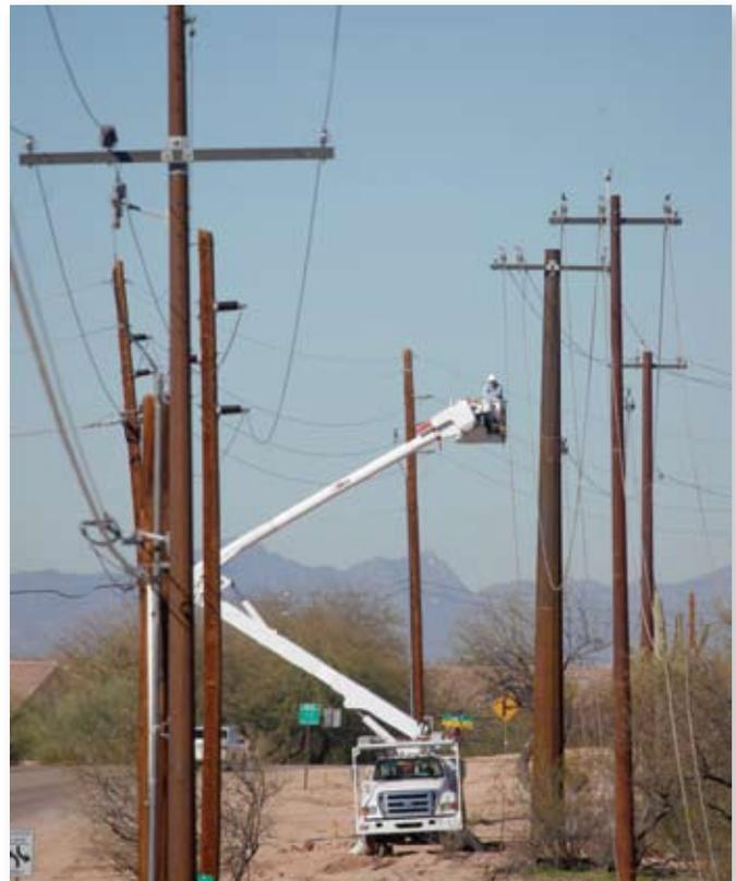
Crews relocate a line because of a road improvement project and use steel for the new poles.
