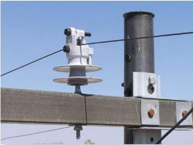
Hendrix polymer vise-top center-phase insulator (shown prior to the raptor hood being installed) is the Tucson Electric Power standard.
