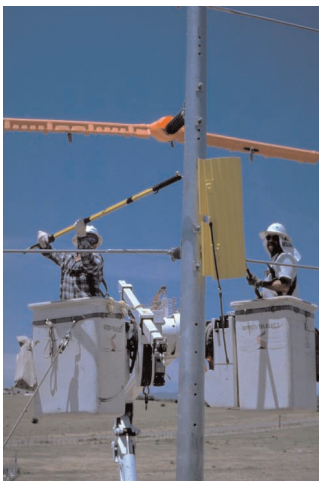
The life span of a steel pole is 60 to 80 years — two times longer than that of an average wood pole.
