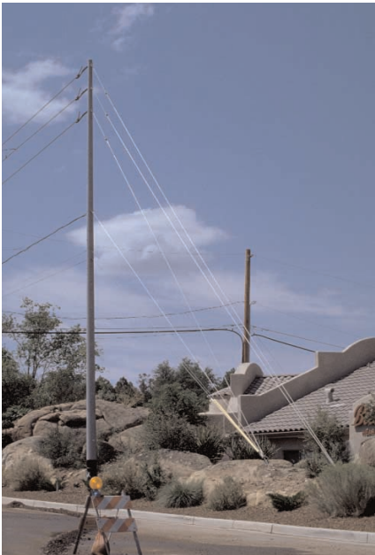
If guying is required, steel poles are guyed using the same hardware currently used for wood poles. Permanent attachments, such as vangs, can be welded into the poles for attaching guys.
