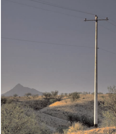
Steel poles are used in all types of environments, from city streets to rolling hills.
