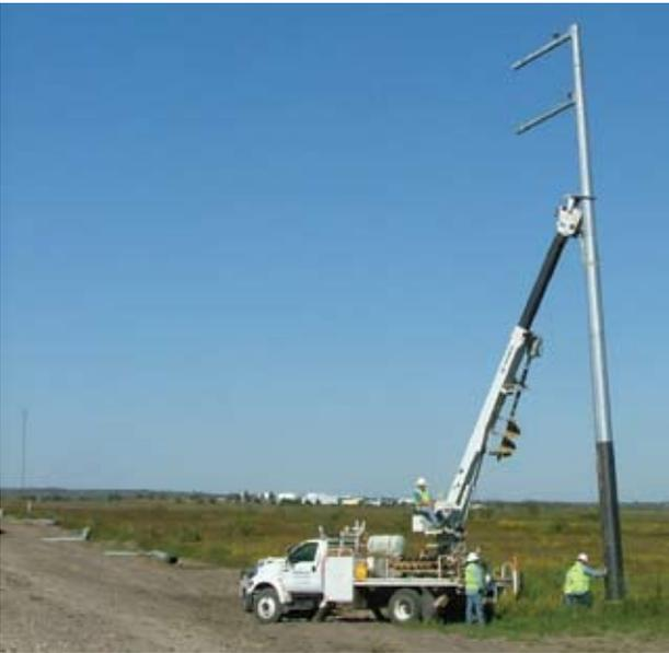
The steel poles may cost more upfront, but Bluebonnet has found that these poles are resistant to decay and woodpecker damage, and with proper maintenance, they will significantly outlast a typical wood pole.
